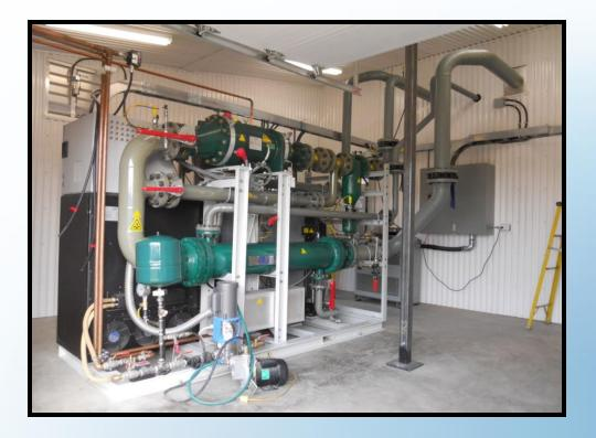
Combustion of wood wastes and recovery of heat to fuel a 100 kWe Organic Rankine Cycle (ORC) CHP system.
