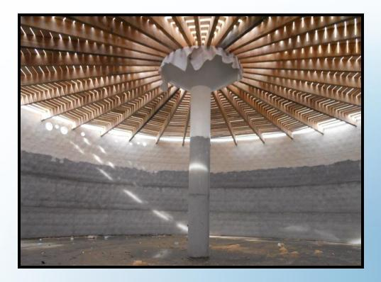
Interior of anaerobic digester. Overhead frame work supports bacteria that feed on hydrogen sulfide.
