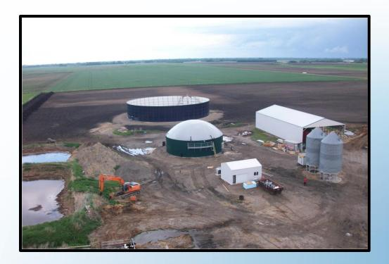
Production of biogas via the anaerobic digestion of organic wastes to fuel a 70 kWe internal combustion engine driven CHP system.
