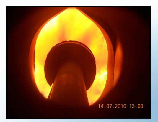
Replacement of heavy fuel oil with pyrolysis oil to fuel a 15 MWe boiler & steam turbine CHP system.
