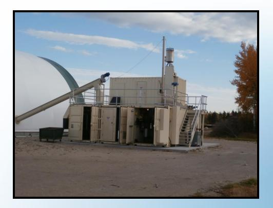
Gasification of wood wastes to fuel a 100 kWe internal combustion engine driven CHP system.
